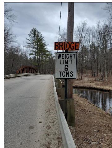
The River Road Bridge in North Weare has been posted with a weight limit of six tons after state inspection (Tom Clow photo).
