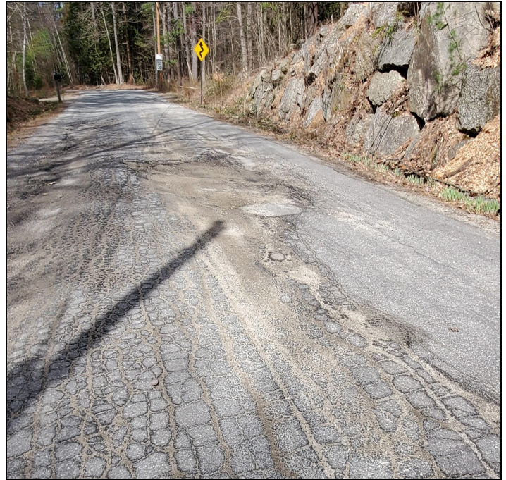
High Rock Road, which shows pavement deterioration and water collecting in the road, will be rebuilt this summer (Tom Clow photo).
