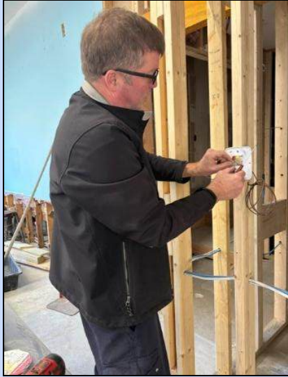
Kevin connecting the heating system donated by Granite State Plumbing & Heating
