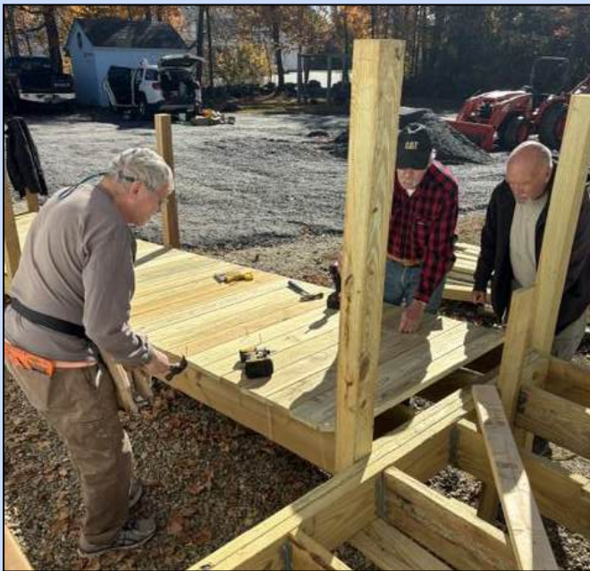
Joe McCarron, Greg Walthers and Mike Pelletier working on the second ramp
