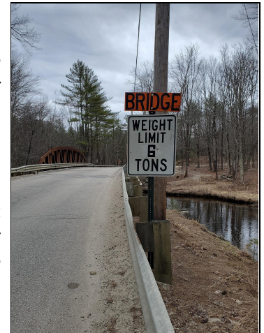
The River Road Bridge in North Weare has been posted with a weight limit of six tons after state inspection (Tom Clow photo).
