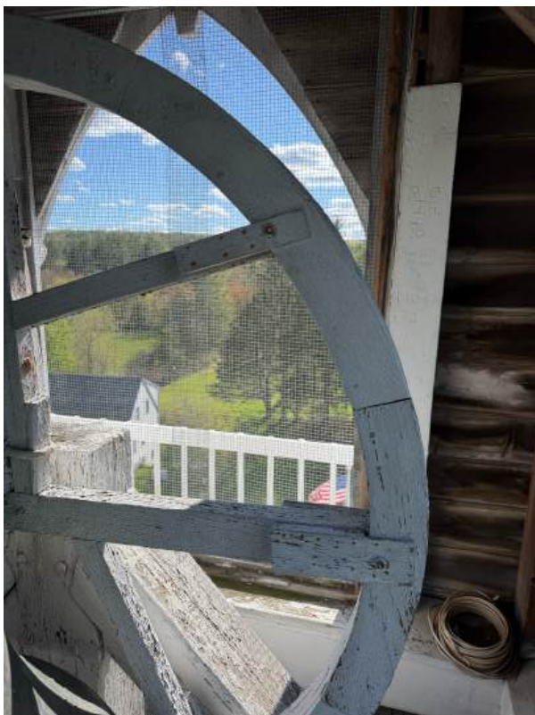
A view from the bell tower of the Old Town Hall is seen here through the spokes of a wagon wheel that is part of the mechanism that rings the bell. A rope is attached to one of the spokes in the wheel and drops through to the second floor. When it is pulled, it turns the wheel and rings the bell. (Courtesy photo)
